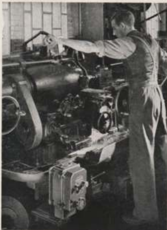
Push-button starter on Capstan Lathe
